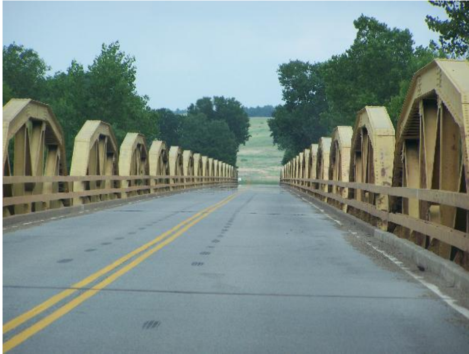
Route 66 Pony Bridge, near Bridgeport, Oklahoma
